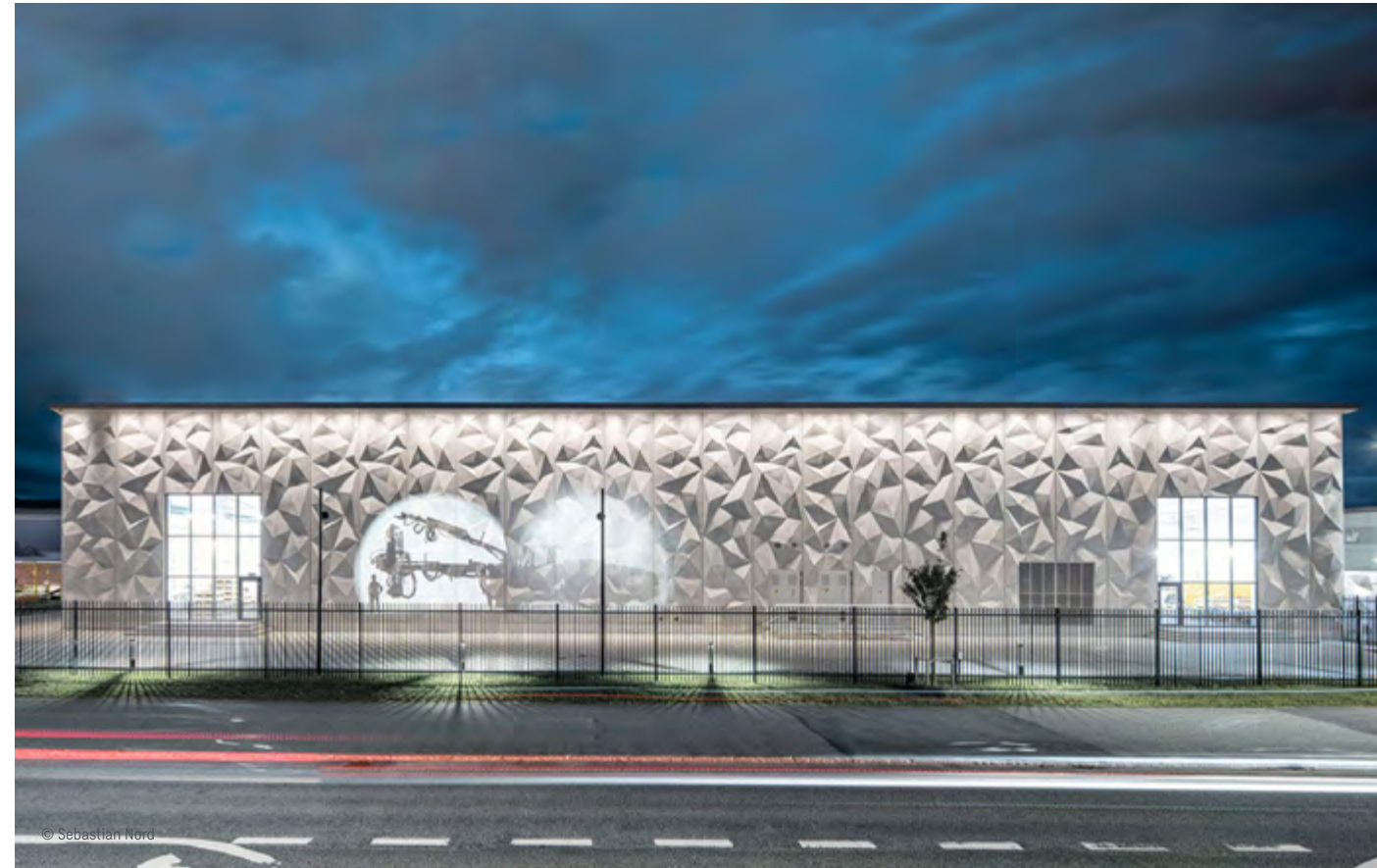
Heat treatment facility Epiroc AB Örebro, Sweden
