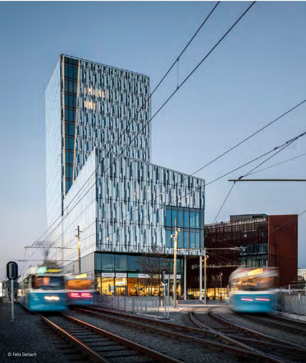
Gamlestaden Station Travel Center Göteborg, Sweden
