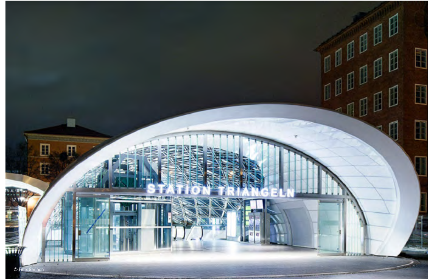
Station Triangeln City-Tunnel Malmö, Sweden
